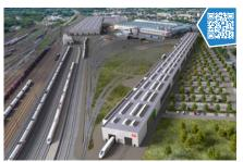
In future, heavy maintenance of the entire ICE 4 fleet of **Deutsche Bahn AG** will be carried out in the new Cottbus maintenance works. The double-track facility in the image's foreground will go into operation in 2024, with the four-track hall at the rear to begin operation in 2026. The existing building in between is used for the maintenance of diesel locomotives.
